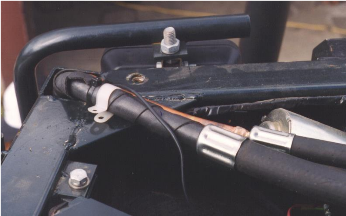
Column lines at top of column with nylon clamp and clutch wire shown.
